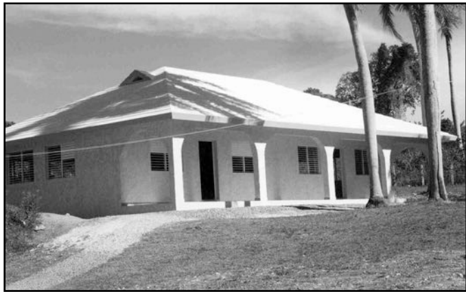
Classroom building — finished — much landscaping needs to be done.
