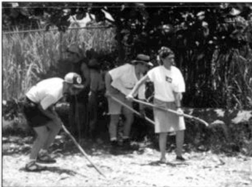
Road construction at the Business School campus.
