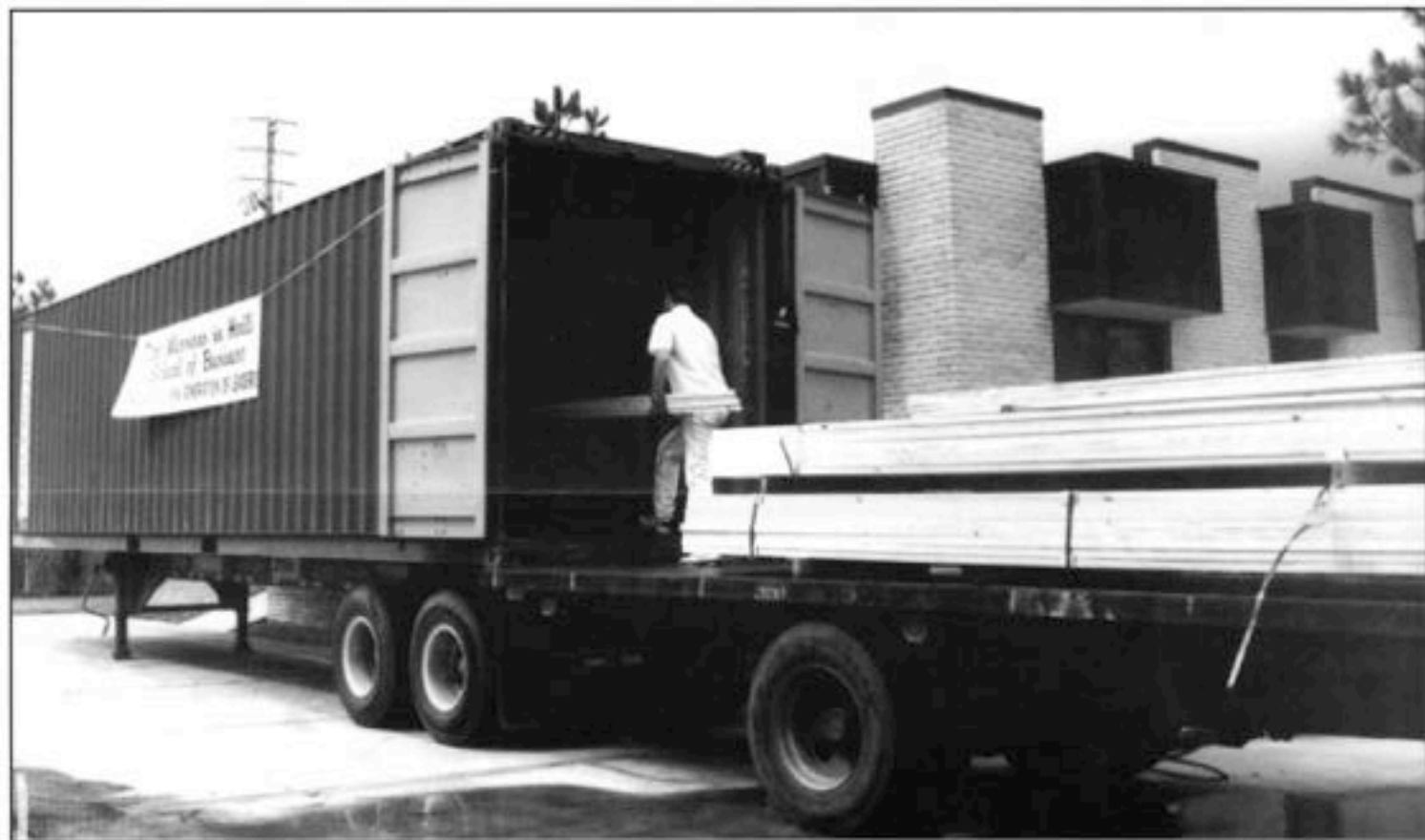
Together we are training a new generation in Haiti. Lumber for the construction of the Business school in Haiti was another priority on the container.
