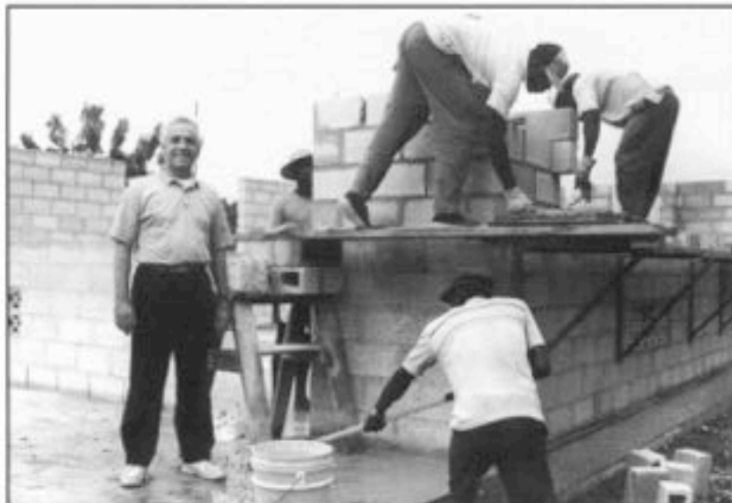
Pastor George at the administration building construction site.
